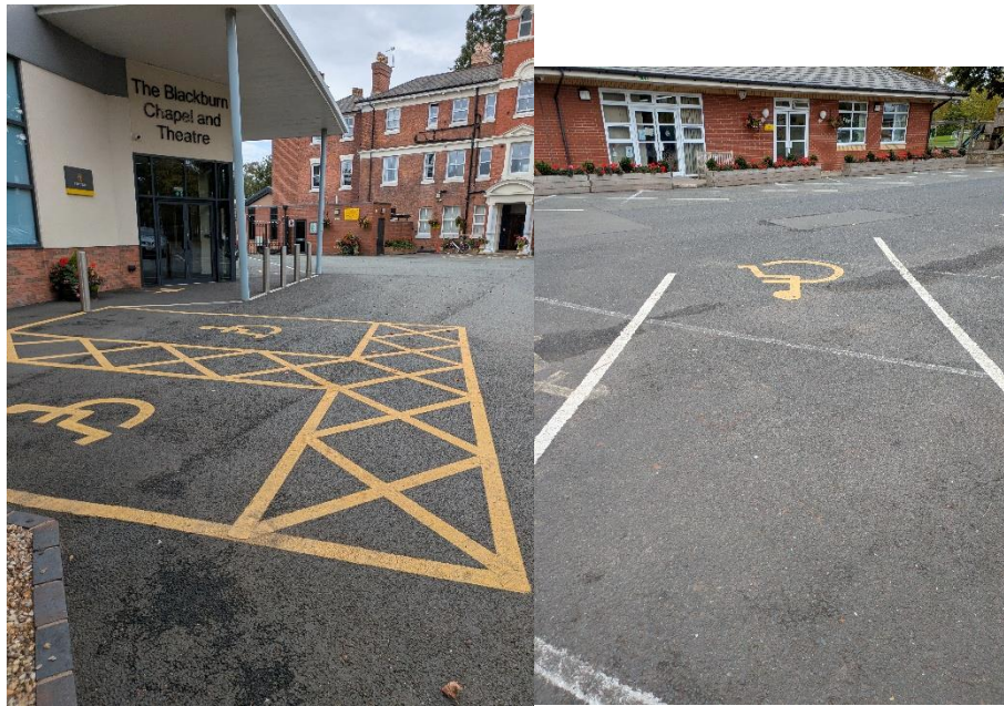
Designated car parking bays. Completed: 2015
