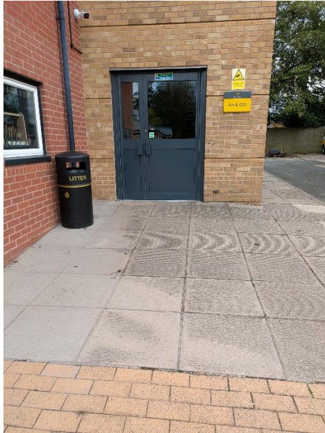
Access to Art and CDT. Completed : 1980s
