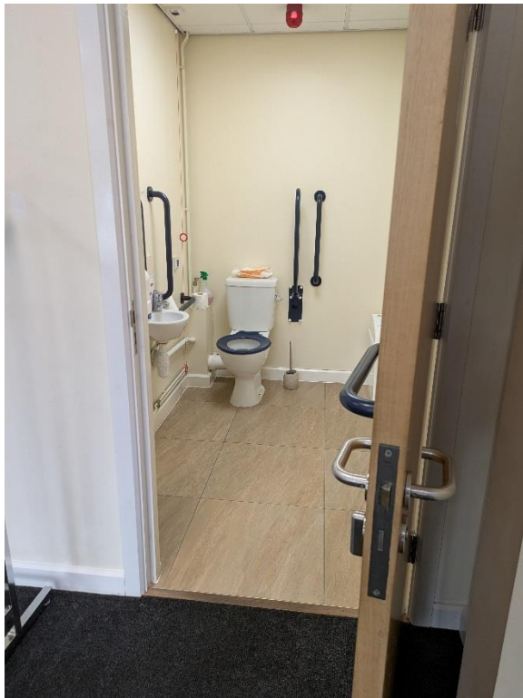
BCAT disabled toilet. 2015
