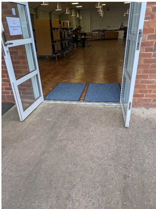
Access to dining hall. Completed 2005
